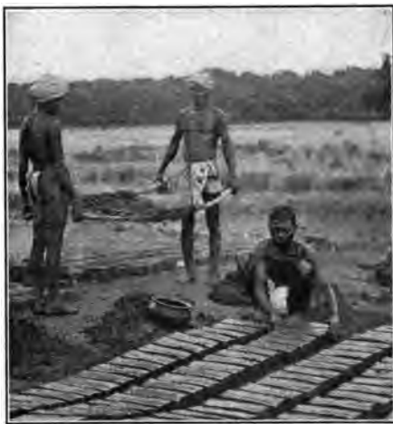
FIG. 120. — Brick making in the old way, India.
